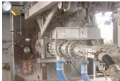
Burner for petcoke, solid wastes, natural gas / diesel oil lance. ( http://www.dynamis-ma.com/ )
